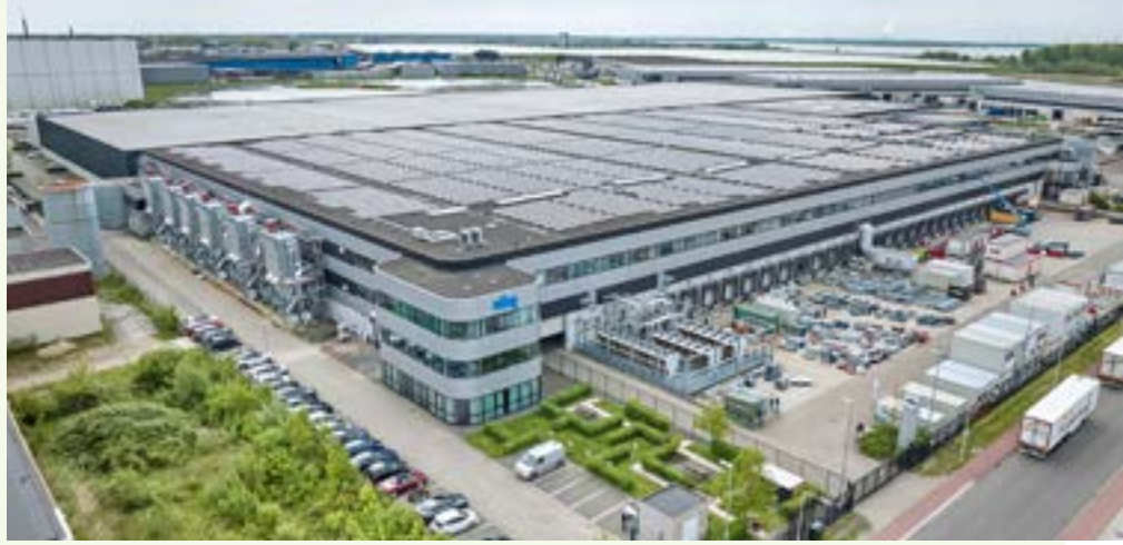
UBQ Facility in Bergen op Zoom, the Netherlands. Source: UBQ
